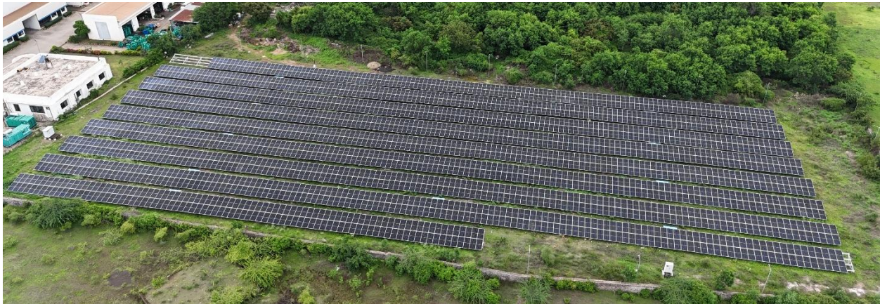
Figure 16. In-House Solar Panels Installation at Lonand
