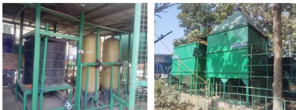
Figure 23. Sewage Treatment Plant
